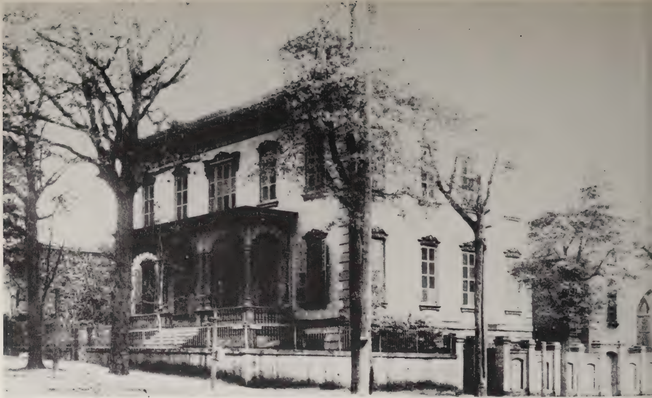
Baldwin home at the SW corner of Perry and Adams Streets has been demolished. (1890)
